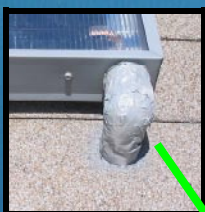
Finished feed assembly with Insulation, aluminum tape and matching paint
